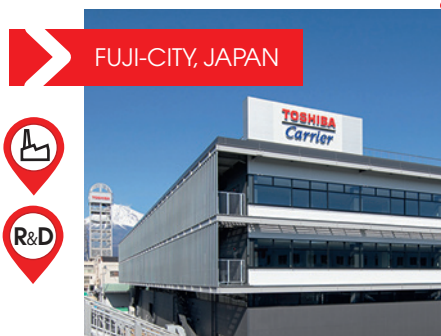
TCC - PRODUCTION FACILITIES and TCC - ENGINEERING CENTRE
