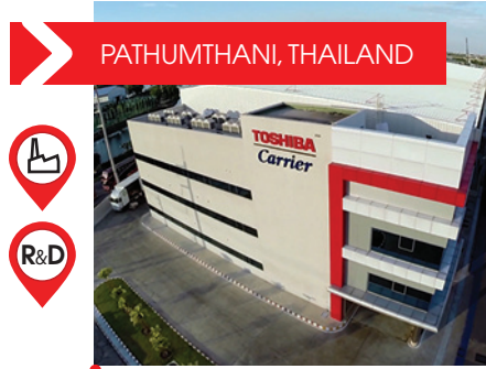
TCTC - ENGINEERING CENTRE
