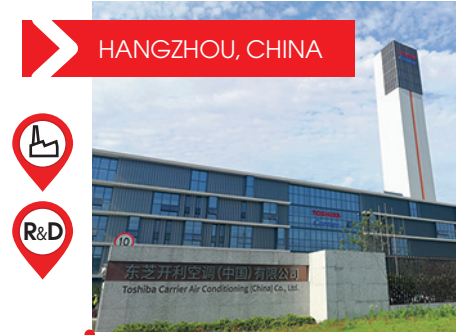
TCAC - PRODUCTION FACILITIES
