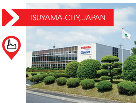
TCC - PRODUCTION FACILITIES
